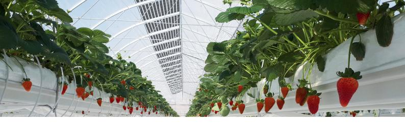
Richel Group positions itself as an essential partner for cultivating crops while generating watts through the photovoltaic poly greenhouse: a diffusing film, flexible positioning of roof panels and an adaptable shading ratio.
